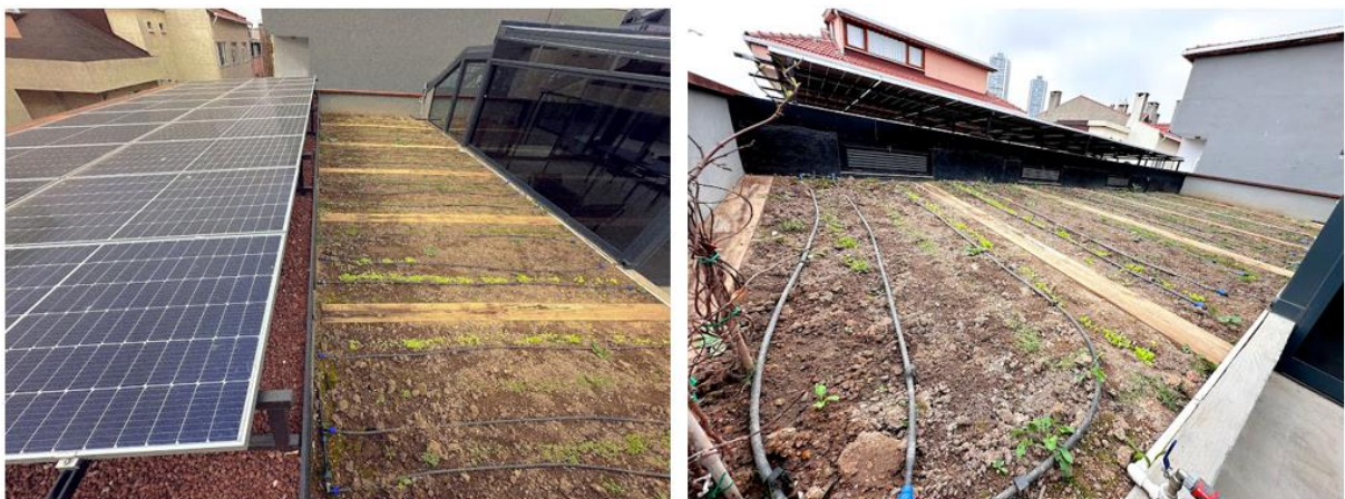
Figure 3: Solar energy panels & sustainable terrace.
