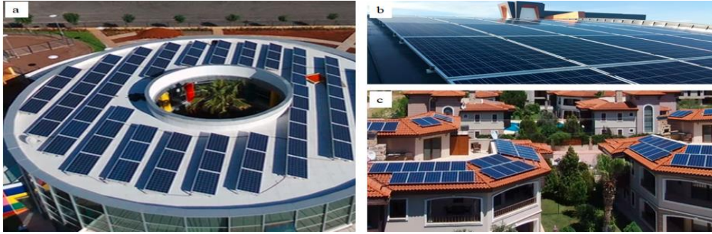
Figure 1: PV panel roof applications; a) terrace roof PV systems, b) integrated PV systems, c) mounted PV systems (Daima Enerji, 2023).
