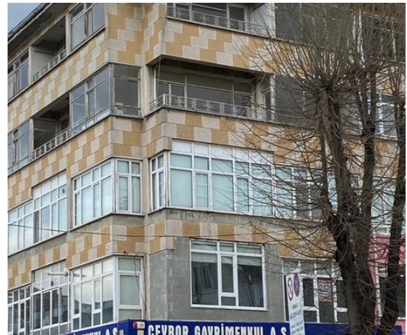
Figure 8: An example where open projections are transformed into enclosed extensions and incorporated into interior spaces (From Esra Bostancıoğlu archive, Adapazarı)
