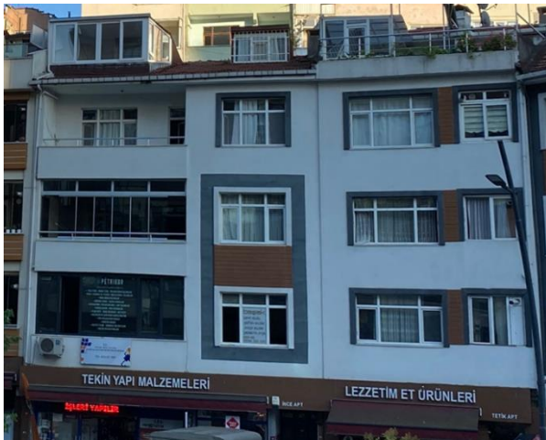
Figure 7: Three independent additional spaces are observed on the roof of the building, with the addition of three separate stairs and the creation of gaps in the slabs (From Bostancıoğlu archive, Istanbul).
