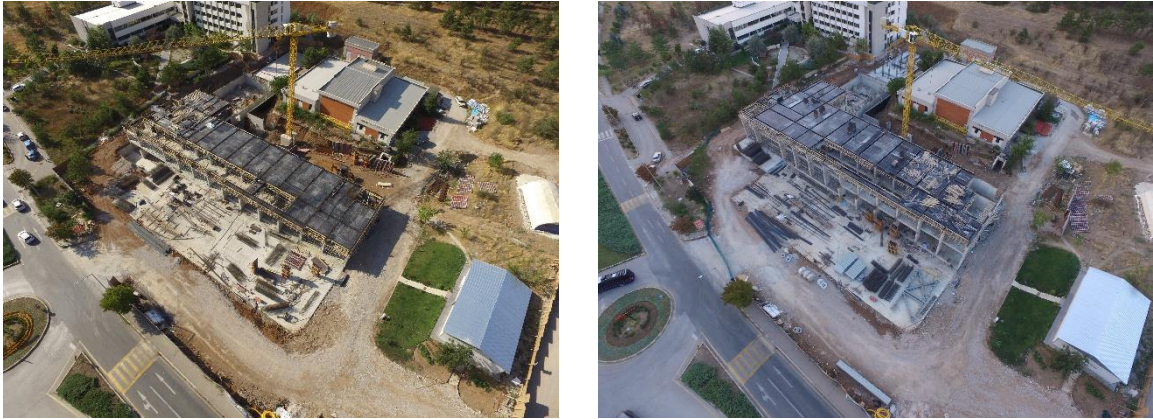
Figure 3: Input images for construction progress tracking.
