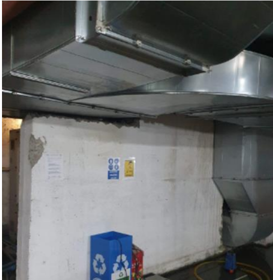
Figure 4: Cut reinforced concrete shear wall at Adiyaman Özel Gözde Medical Center (Example of structural element intervention) (ITU, 2023).
