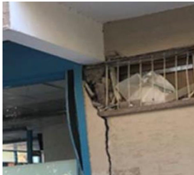
Figure 5: Damage to band windows in a building during the 2020 Izmir Earthquake (IMO, 2020).
