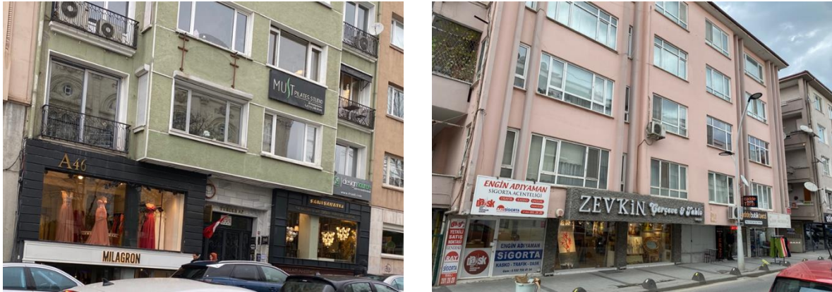
Figure 2: Examples of the removal of infill walls due to the conversion of basement floors into shops (from Esra Bostancıoğlu archive, Adapazarı).
