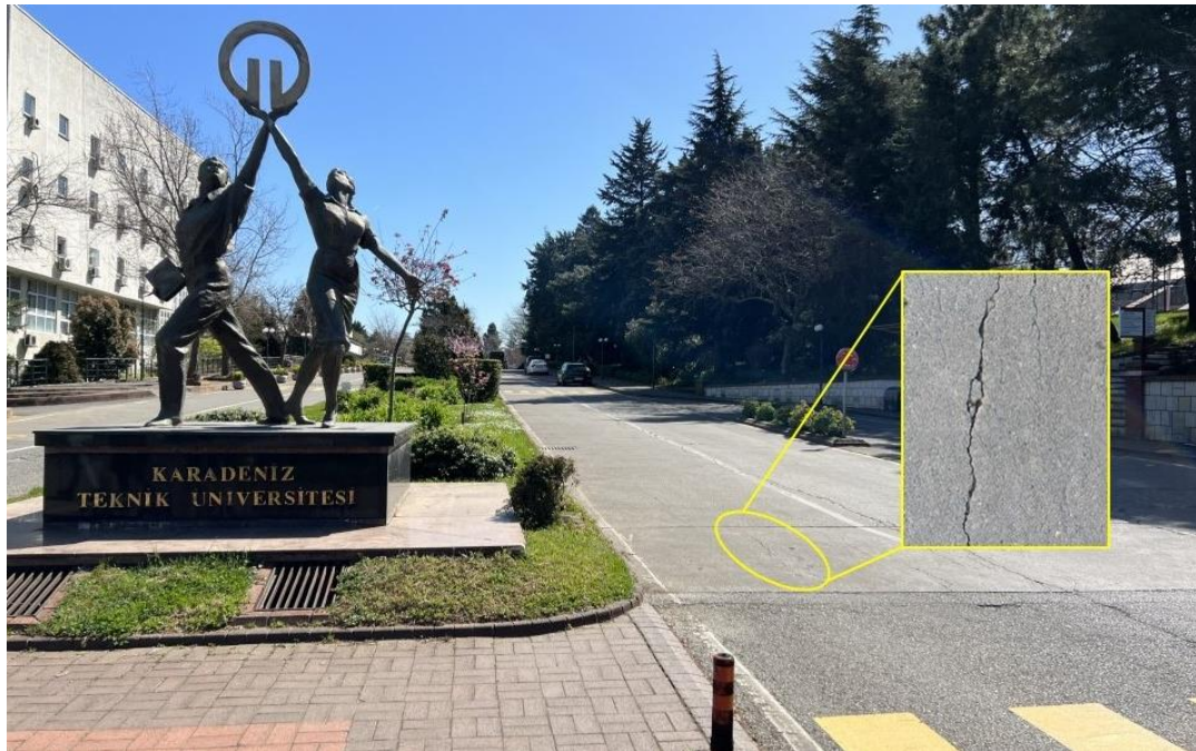
Figure 2: Sampling of crack images obtained from the roads in Karadeniz Technical University Campus.
