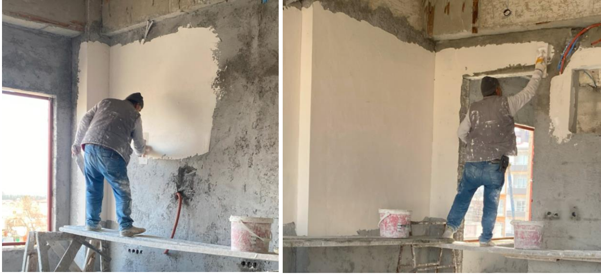
Figure 2: Data collection with sensor attached to the gypsum plaster workers' arm.
